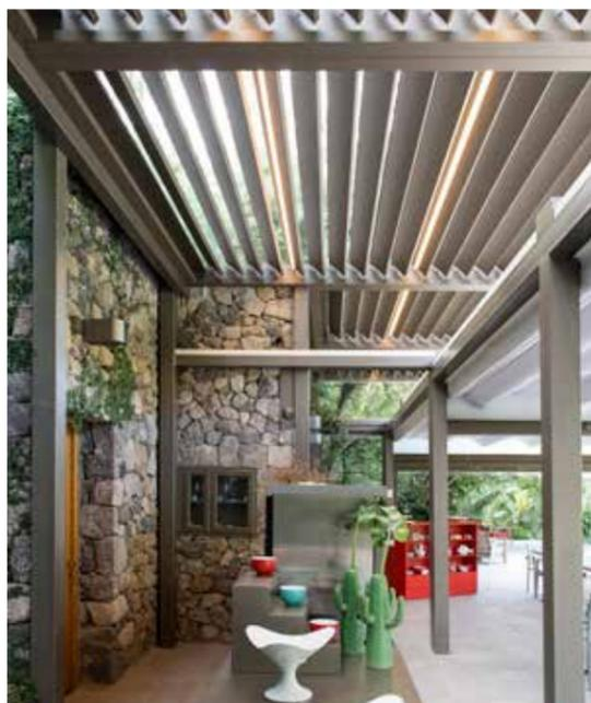
Alba is a bioclimatic pergola fitted with aluminum blades that can be oriented up to 150° using a wireless control to adjust light and ventilation.
